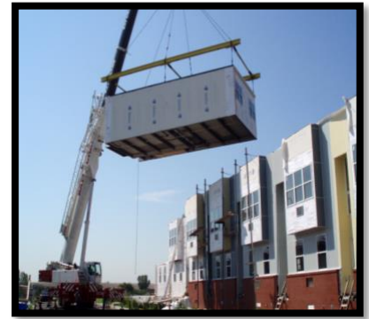
Public housing construction. Portland, Oregon
